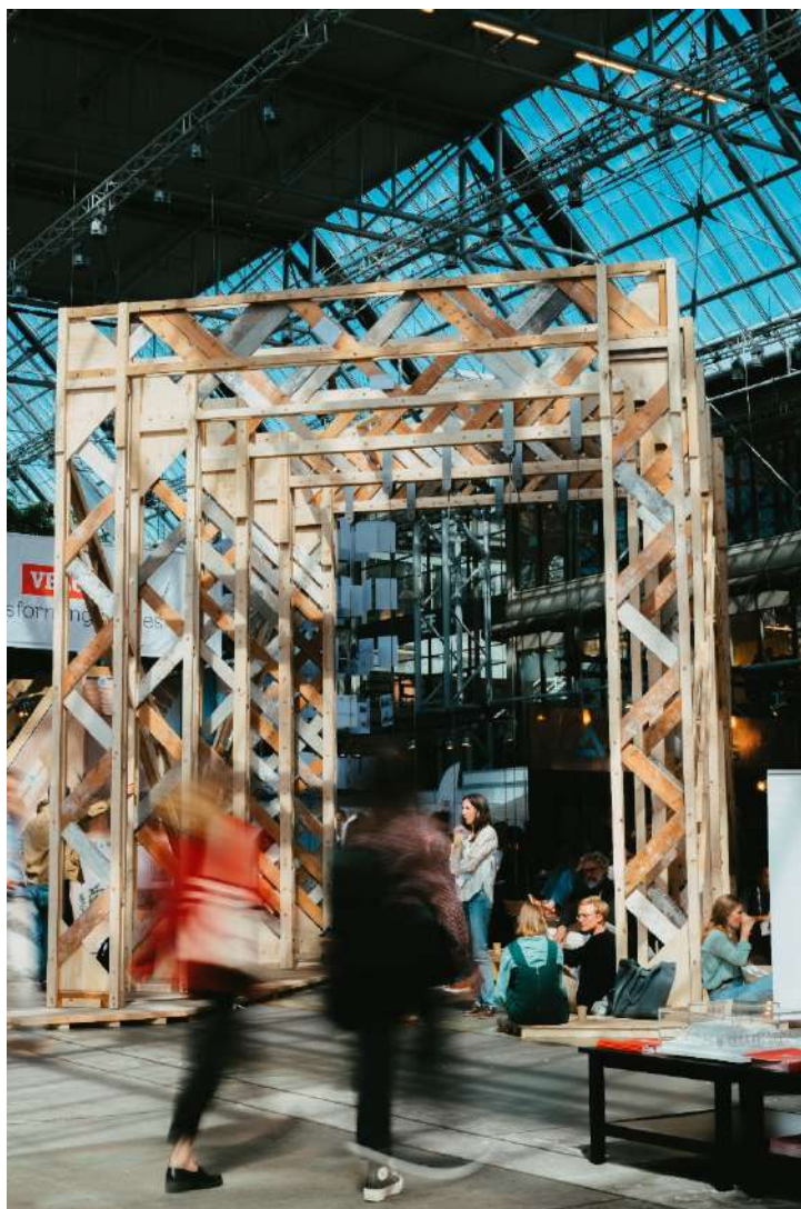
Figure 5: Completed pavilion structure with 5 frames and a hanging amphitheatre.
