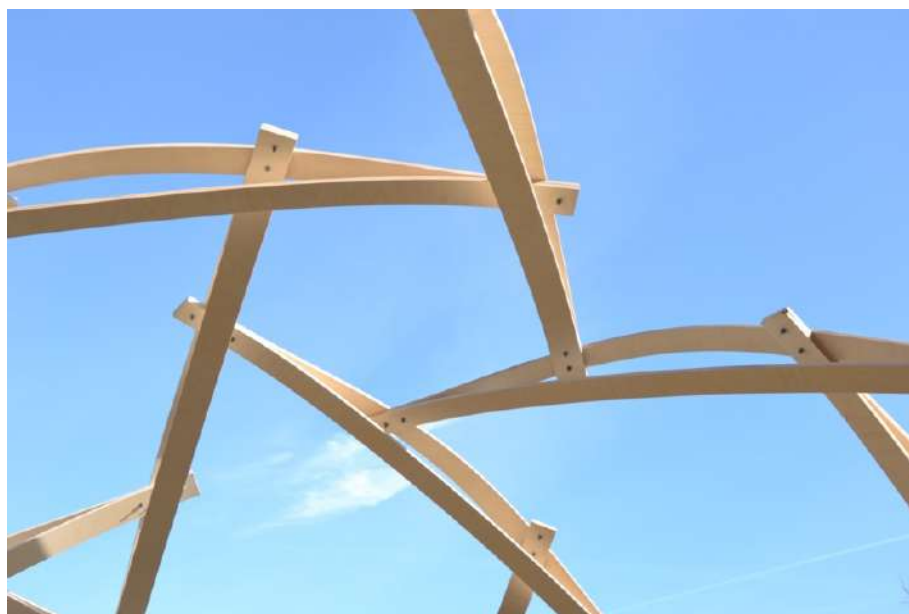
Figure 2: The ReciPlyDome pavilion was built with bending active plywood beams
