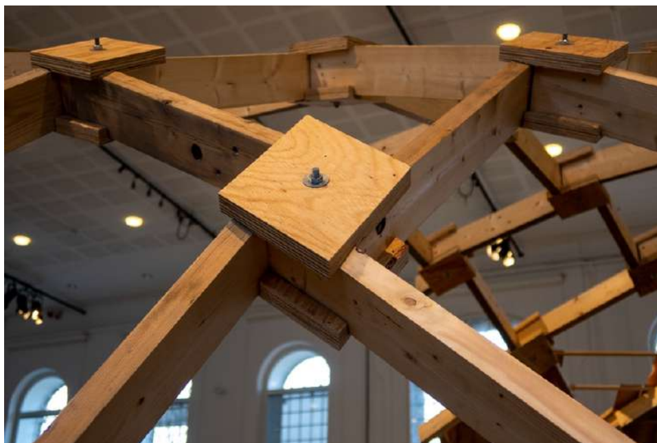
Figure 4: The WasteWood Canopy's clamp connections rely on a single bolt connection,
