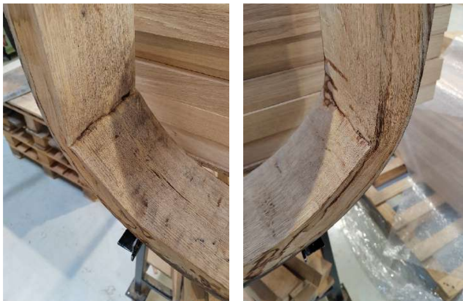
Figure 10 and 11: Collapsed structure of specimens in places of small bending radius
